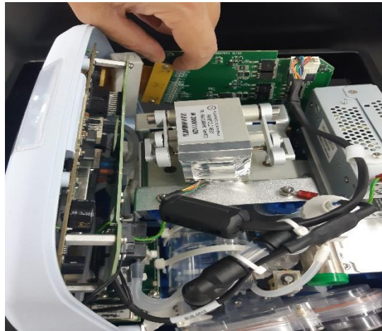
Figure 30 – Flat Flex Cable going to P16
